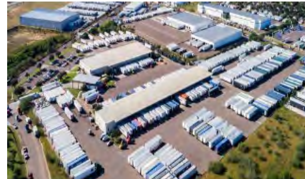
High-flow through truck terminal
