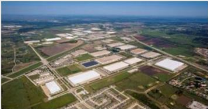
Alliance Texas – Industrial, Fort Worth, Texas
