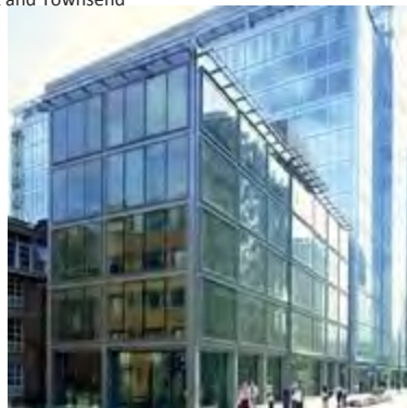
288 Bishopsgate Recently the subject of a mezzanine finance deal
