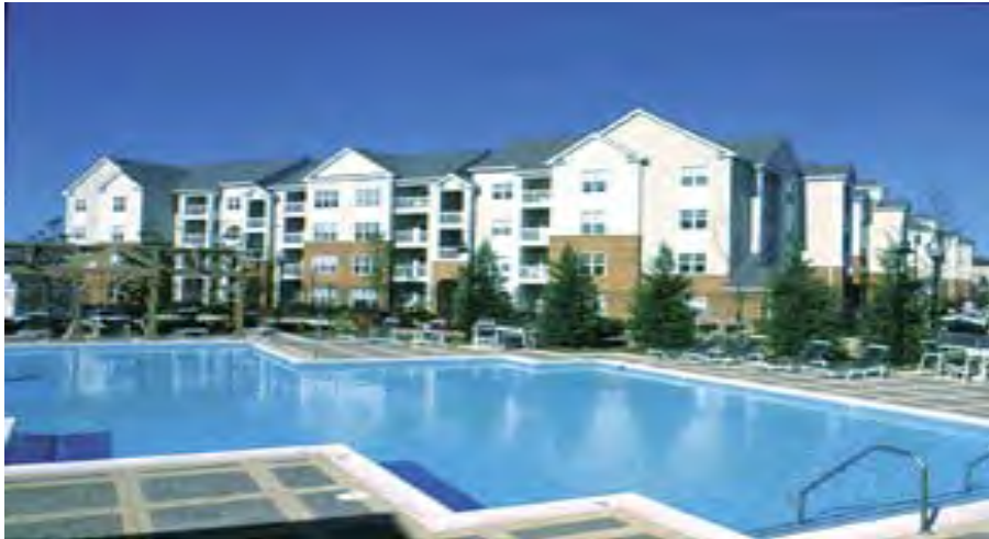
Springfield Station, Springfield, VA
