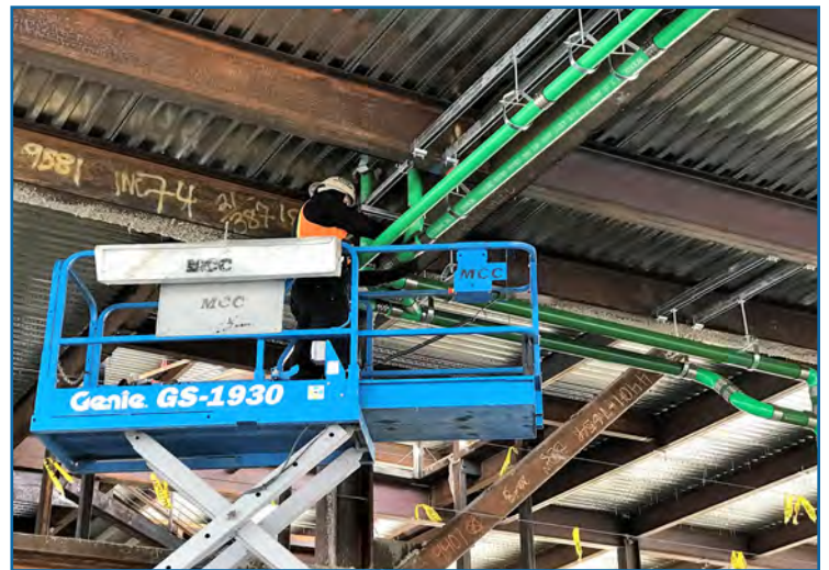
MCC continues rough-in of roof drain piping
