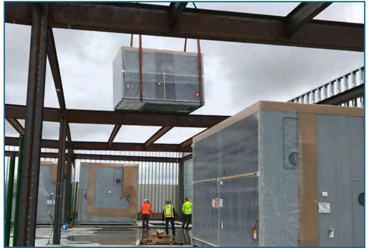
Hoisting section one of five for air handler #3 into the penthouse
