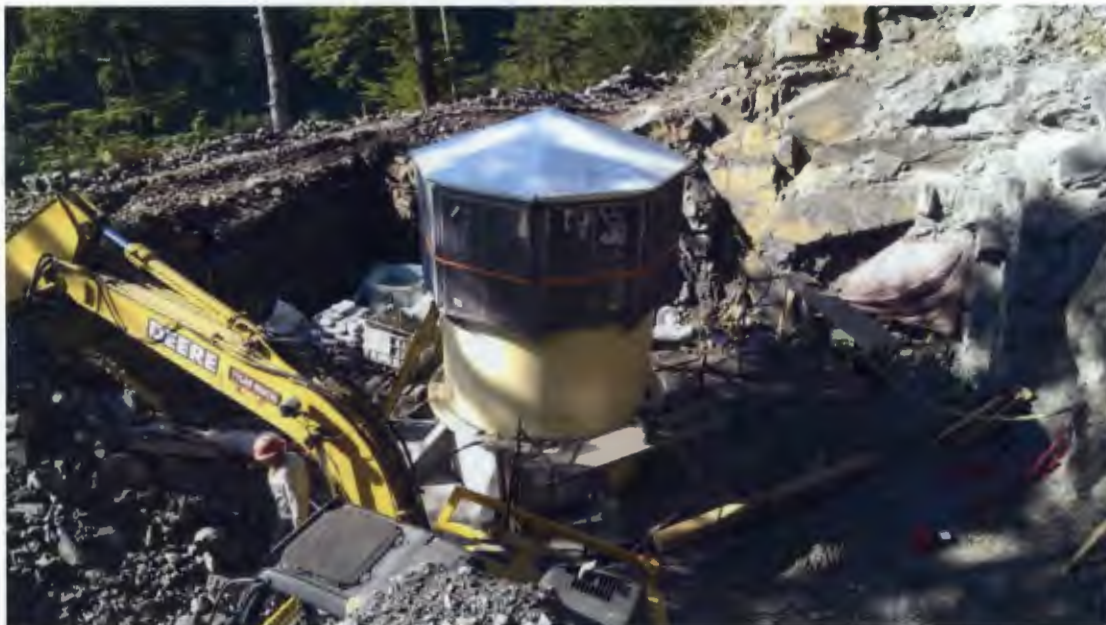
Figure 3: Surge Shaft Top Structure
