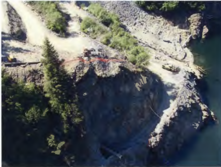
Figure 2: Aerial View of Intake Tunnel Portal
