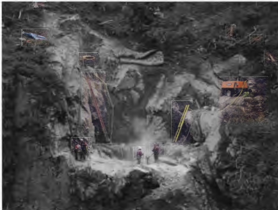
Figure 1: Left Abutment Excavation
