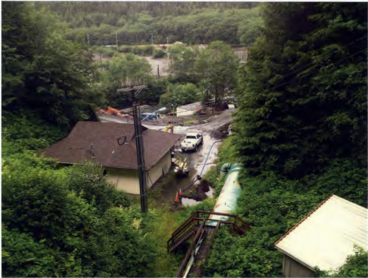
Figure 7. Lower Portal Area, No change this month.
