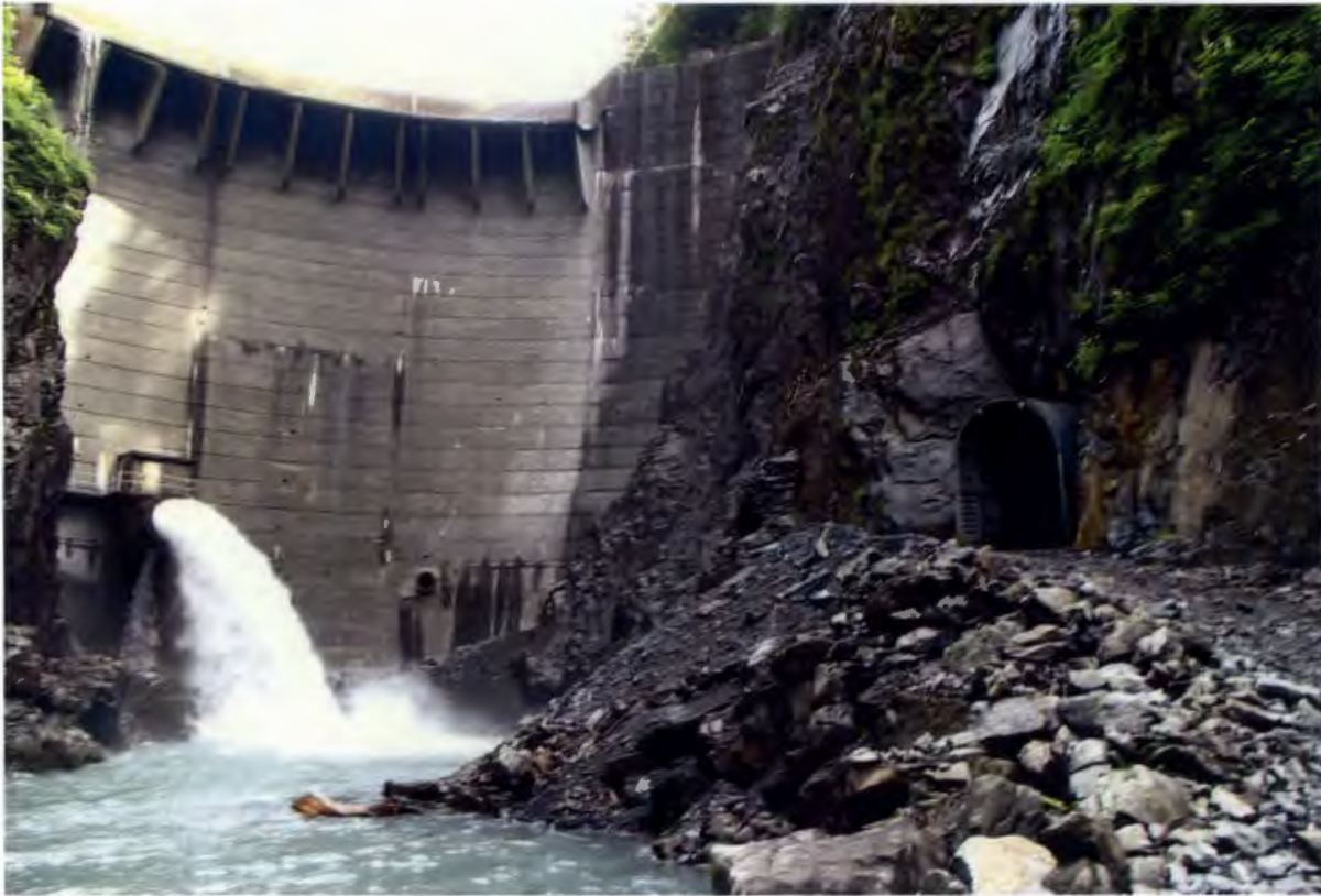
Figure 2. Drainage Tunnel and Scour Wall, the Howell Bunger valve was opened to 10% to control the rising lake level.
